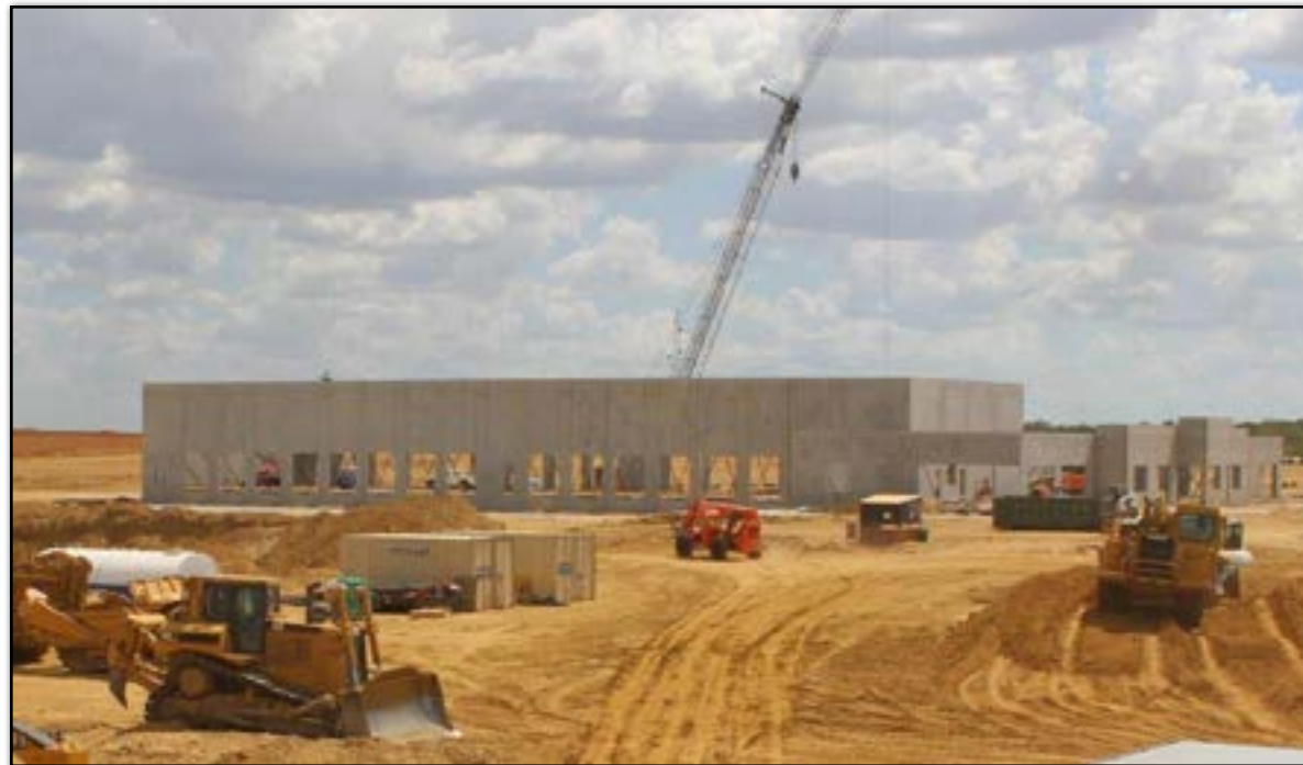
Landstar's Cross Border Logistics Center being built in Laredo, Texas
